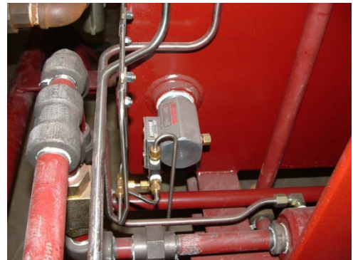
DB40-0400 Air Operated Float Switch (Shown) DB40-0500 Electric Float Switch
